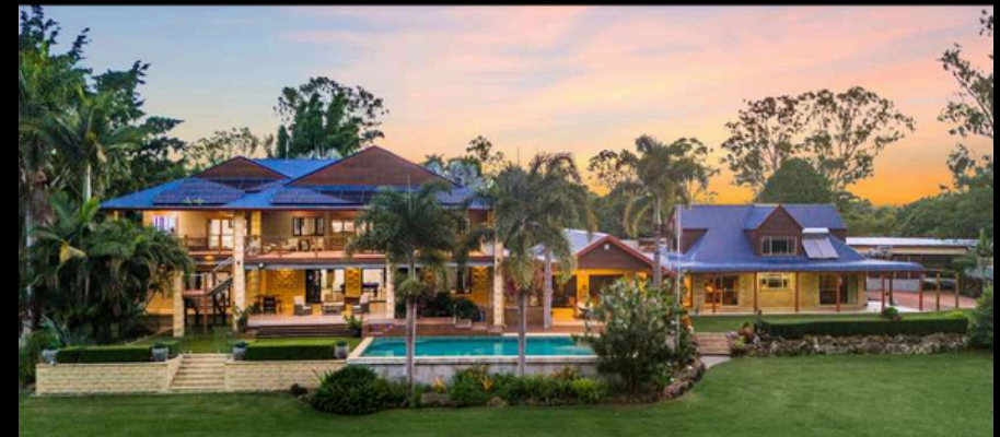
Homestead with function centre and other guest accommodation
